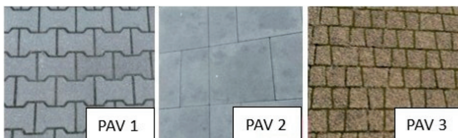
Fig. 3. Types of surfaces used in the tests: PAV 1 – "bone" paving stones, PAV 2 – 0.6 × 0.6 m slab, PAV 3 – piccolino stones
